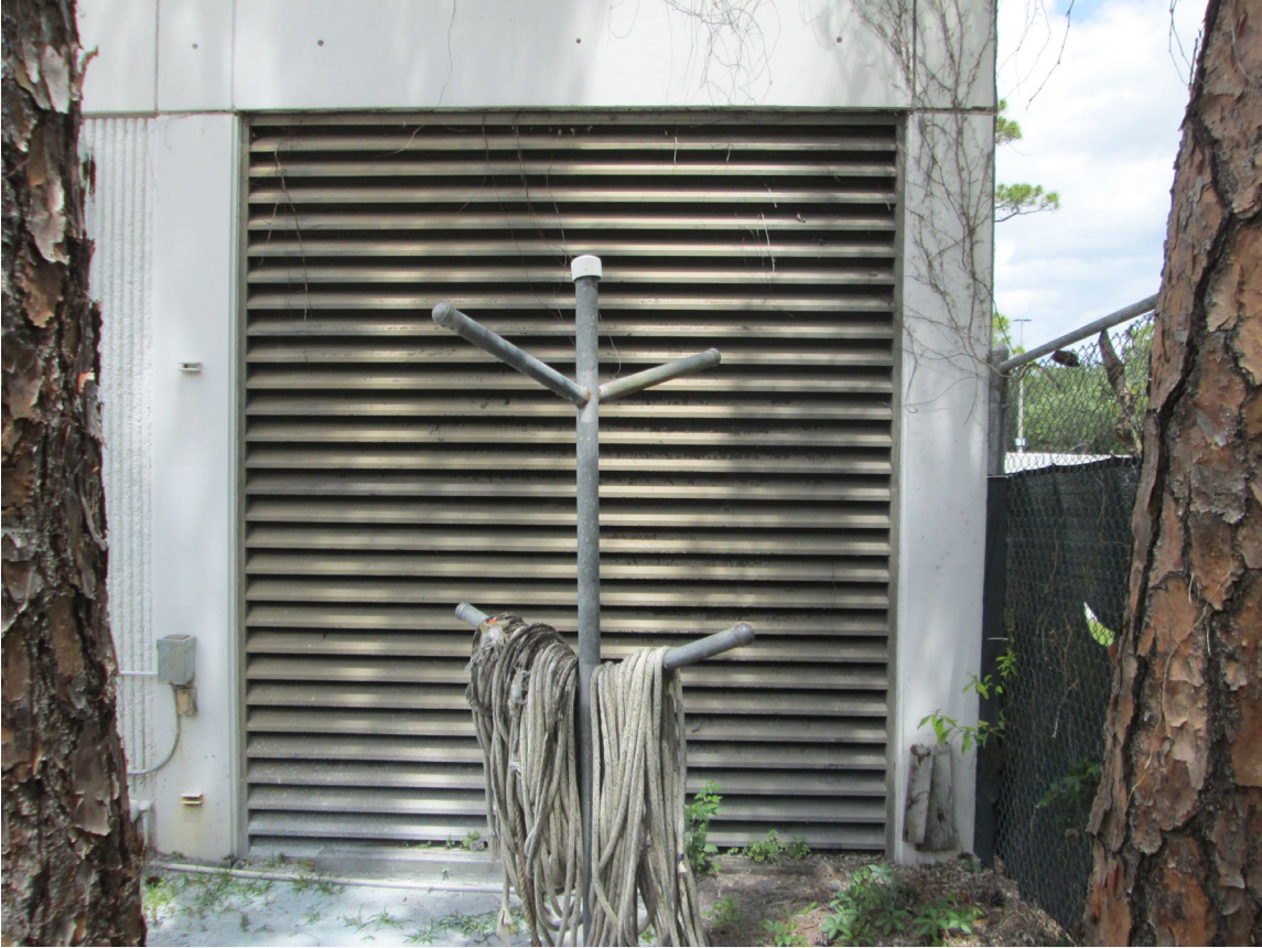
Existing Louvers and Doors are not hurricane-rated
